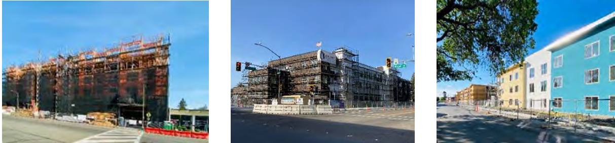
Figure 7 – Multi-family residential projects under construction in downtown Santa Rosa.
